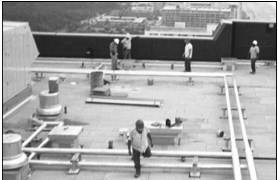
Installing LIGHTGUARD® on Margate Towers in Myrtle Beach, South Carolina.
